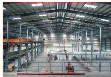
Industrial Work Shop
